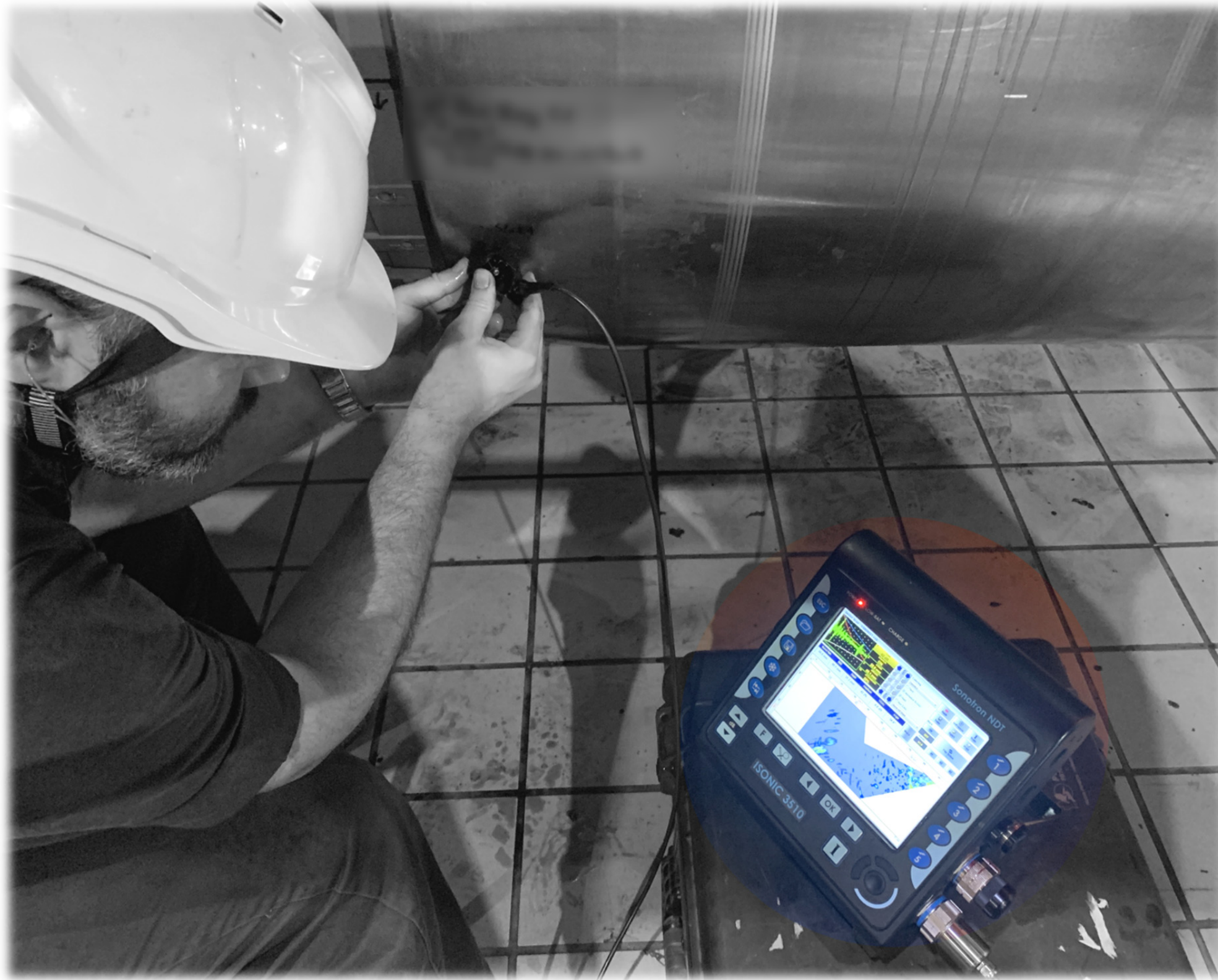
Crack on the ID Surface of Retainer Ring
